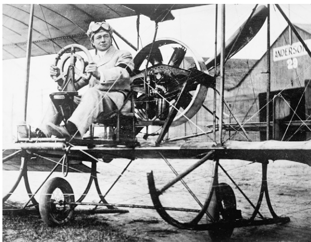
Inventor-entrepreneur Emile Berliner (1851–1929) made a fortune with his improvements to the telephone and phonograph. He was also a pioneer in aeronautical engineering. This photo (ca. 1911) shows aviator Paul Peck at the controls of a helicopter Berliner designed. Photo: Library of Congress.
